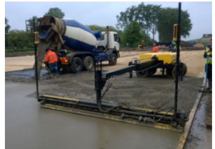
Laser guided screed
