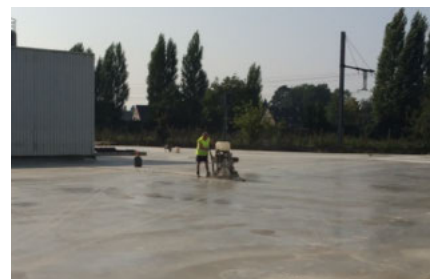
Applying saw cuts
