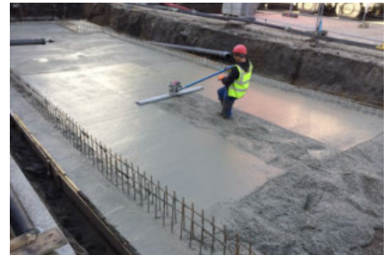
Use a flat skip float to finish SCC
