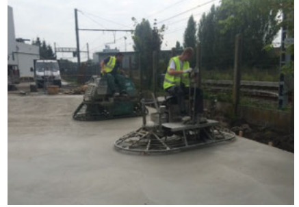
Power floating concrete
