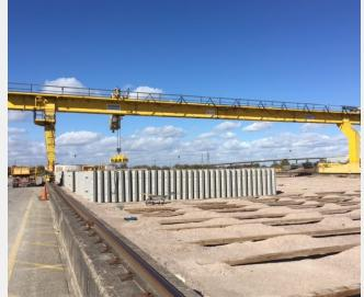
Precast tunnel segments ready for transport to site and installation to provide the tunnel lining of the Northern Line Extension.
