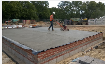
Powerfloat finish is easily achieved with DURUS S400.
