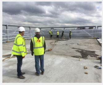
The use of DURUS \$400 allows large areas to be flood poured without any risk of disturbing in-situ steel mesh reinforcement. Insufficient concrete cover is also not a factor as the reinforcement comes ready mixed in the concrete ,which can be easily pumped into position.
