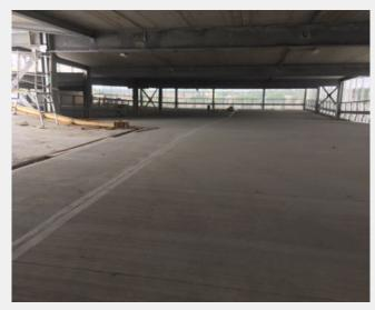
Owing to the confined working area, the handling cutting and fixing of steel mesh would present significant health & safety hazards during installation of the topping, and would also be very time consuming.
