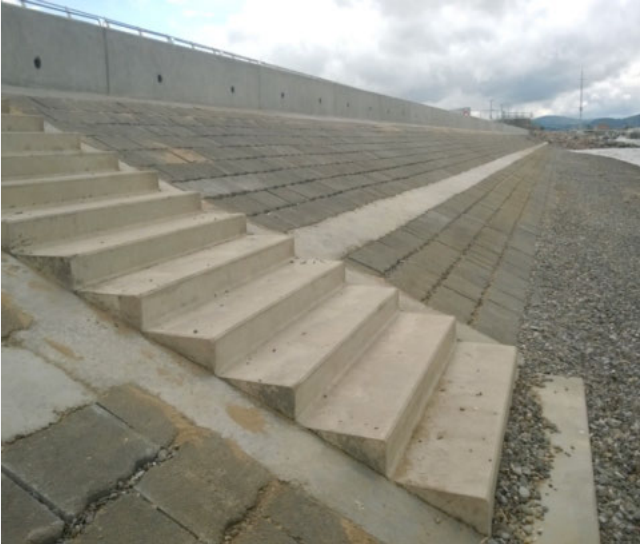
Fibre was used in the construction of the steps too.
