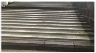
Some of the original Stone Masonary is reused with the remaining concrete channels installed with a Fibre Mix.
