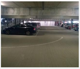
A brush finish was given to the Screed Topping. The Client was very happy with the aesthetics and consistency of the finished surface.
