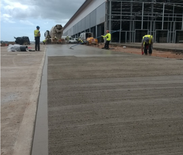
By eliminating steel mesh, large areas can be poured/finished, with saw cut contraction joints being made the following day.
