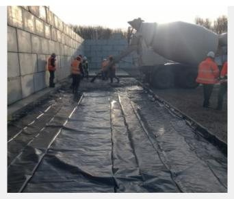
With the **DURUS \$400** Synthetic Macro Fibre reinforcement already contained in the concrete when it is delivered to site, large areas can be poured which greatly reduces construction. Saw cut contraction joints can then be cut 1/3 of slab depth, within 24hrs of placement and finishing.
