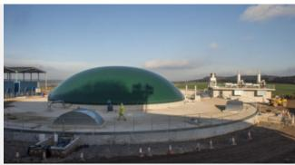
One of the 48m diameter Tanks in which the silage is broken down to produce gas fuel which is burnt to heat water. The resulting steam powers turbines to make electricity.
