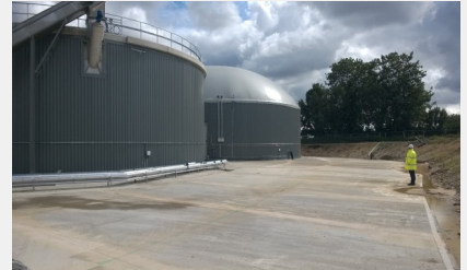
Anaerobic digester facility
