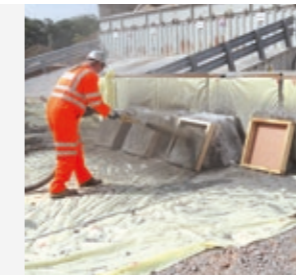
Sprayed concrete
