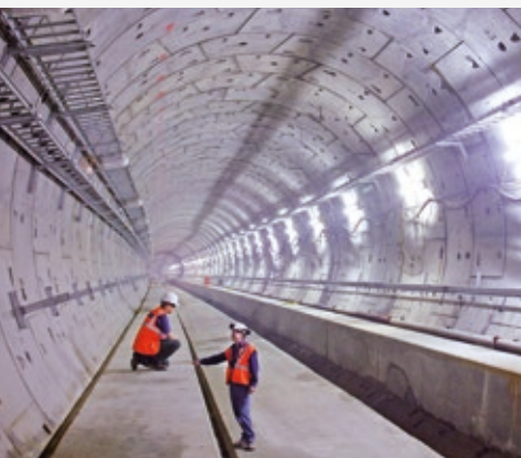
North Downs Tunnel, Kent
