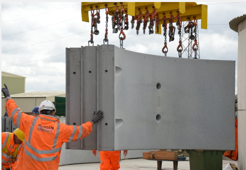
Trial precast segmental lining elements reinforced solely with Durus S500
