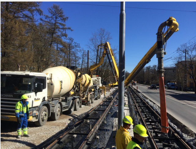
Tallinn Tramline project during installation of Durus EasyFinish fibre reinforced concrete.
