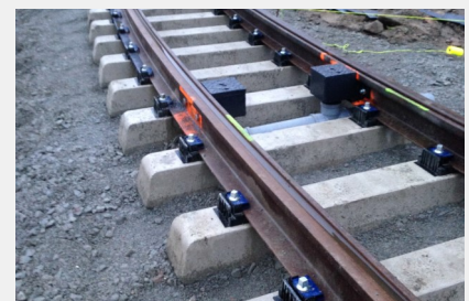
Track slab - Belgium
