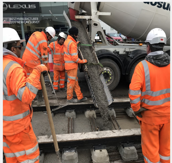
Durus EasyFinish MFRC can be poured directly into place without the need for complicated cutting and fixing of conventional steel mesh.
