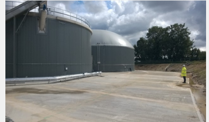
Anaerobic digester facility
