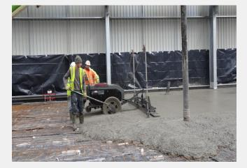
A laser screed could be used continuously without the need for breaks in installation to fix a top layer of conventional steel mesh reinforcement.
