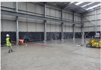
Large areas of pavement could be poured and power floated. Saw cut contraction joints were then made the following day.
