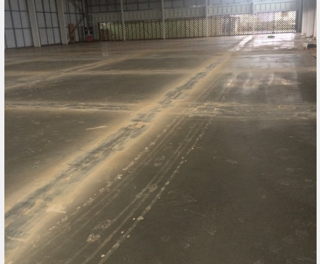
Large areas of pavement could be poured and power floated. Saw cut contraction joints were then made the following day.
