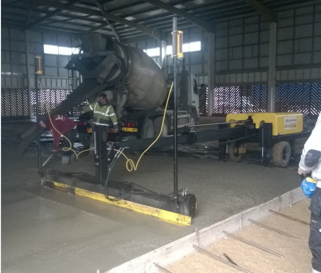
A laser screed could be used continuously without the need for breaks in installation to fix conventional steel mesh reinforcement.
