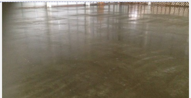
A high quality power float finish was achieved using DURUS S400 Synthetic Macro Fibres.
