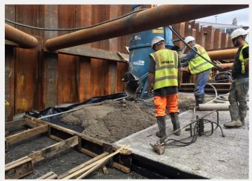
The confined nature of the site would make it difficult and dangerous to handle, cut and fix welded steel fabric. The DURUS \$400 Macro Synthetic Fibre Reinforcement is contained within the concrete on delivery, so cannot be placed incorrectly or disturbed during installation.
