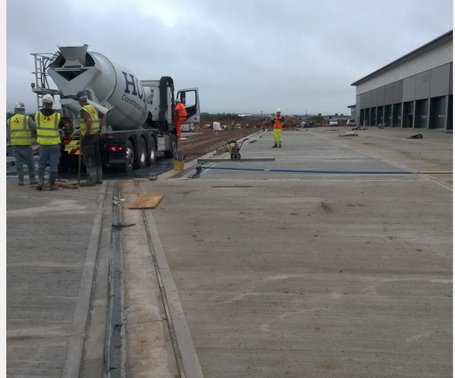
As the reinforcement is dosed into the concrete during batching, the mixer truck can discharge directly into the formwork.
