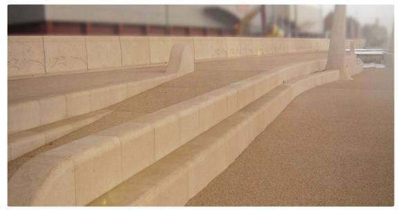
Figure 4 right: Ovingdean and Brighton Marina sea wall and ramp containing Fibrin Fibres.
