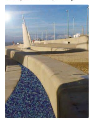
Figure 1: Blackpool Wave wall, berm slab and revetment.
