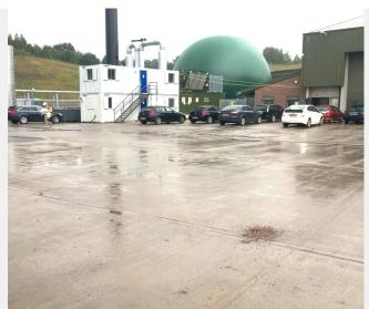
Large areas of pavement could be poured and then saw cut contraction joints made, without delays from steel fixing
