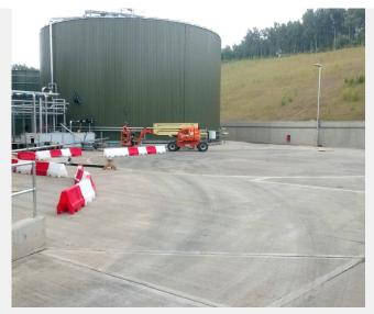
Acidic organic waste is stored in large fermenter tanks before the gas is drawn off; the risk of corrosion in this area is now eliminated
